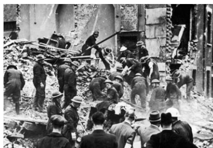
Demolition in Bermondsey after WW2 reveals an unexploded bomb
