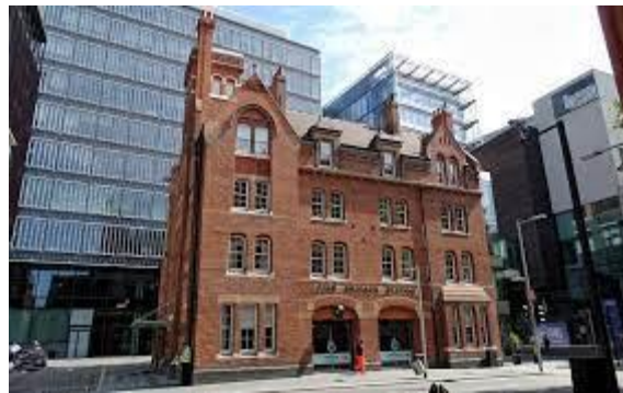
Fire station building (now Brigade restaurant)
