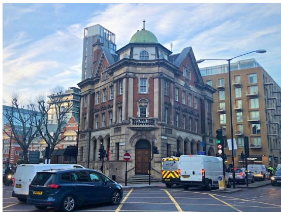
The bank building
