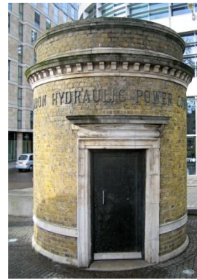
The entrance on the north bank
