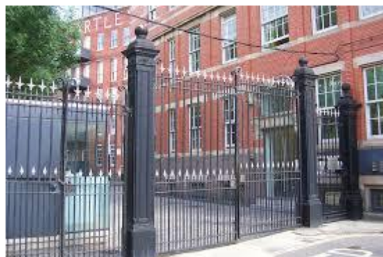
The gates after refurbishment
