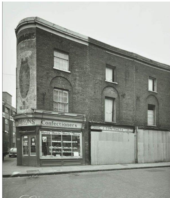
The shop as seen from the west side of Bermondsey Street
